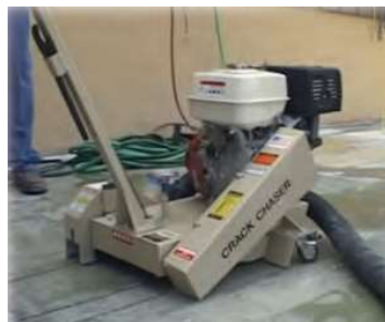
EDCO C10 8" CRACK REPAIR SAW
